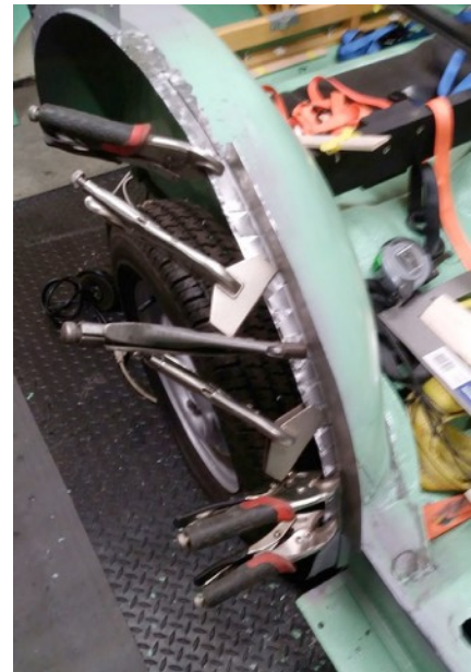
Prepping for welding on repair section.
